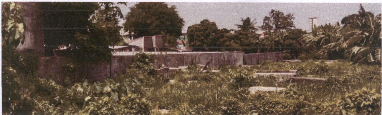
Figure 2. Wall delineating the boundary between the cemetery and subject property
