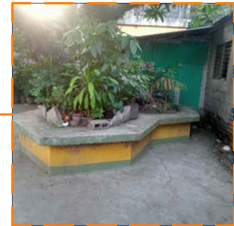
BENCH REPAIR AND REPAINTING
