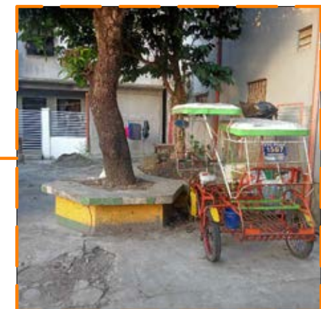
BENCH REPAIR AND REPAINTING
