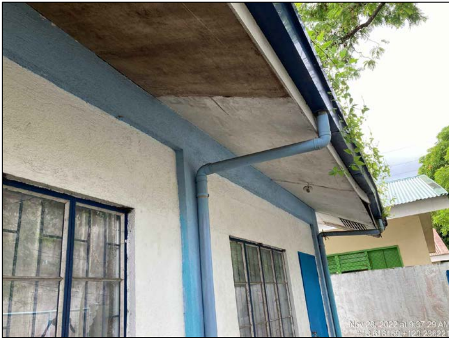
REPLACEMENT OF DAMAGED CEILING ESTIMATED AREA = 40.00 sq.m.
