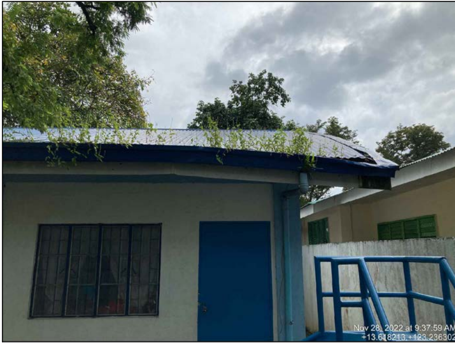
REPLACEMENT OF DAMAGED ROOFING & ROOF FRAMING ESTIMATED AREA = 28.00 sq.m.
